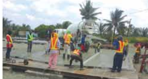
■ On-site Reinforced Concrete Panel Casting
