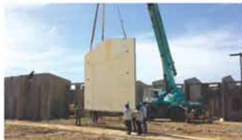
■ Precast Panel Installation
