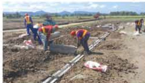
■ Precast Reinforced Concrete Grade Beam Foundation Laying
