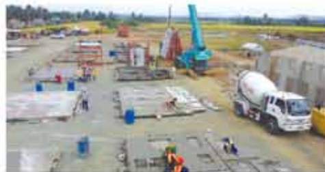
■ Woodendragon's On-site Precast Reinforced Concrete Panel Production Yard
