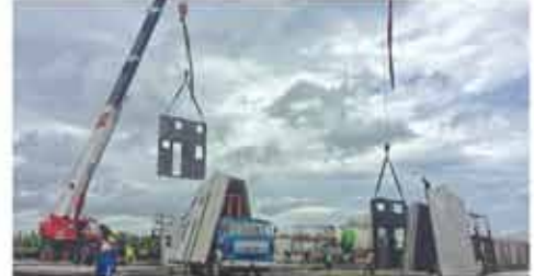
■ Precast Panel Truck Loading and Stacking
